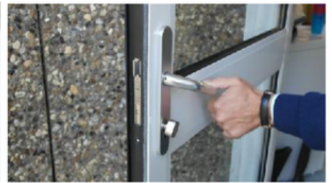
In means of escape door will unlock when handle is operated internally
