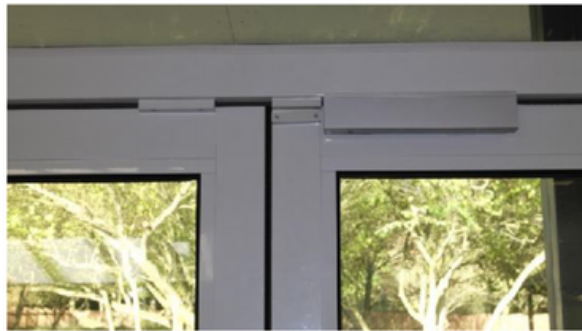
In means of escape door will unlock when handle is operated internally
